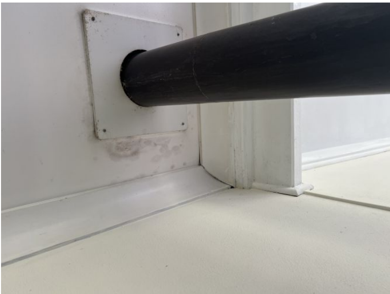
Image comments: Water marks around flue
