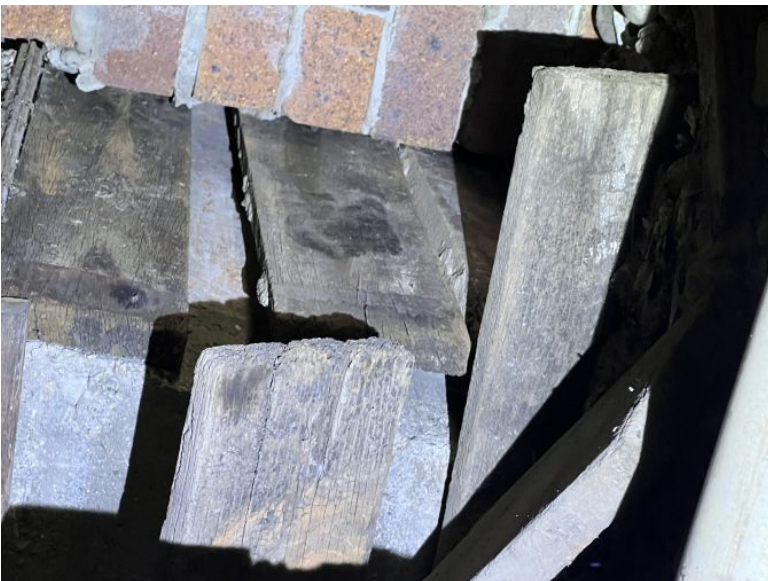
Image comments: Formwork still in position
