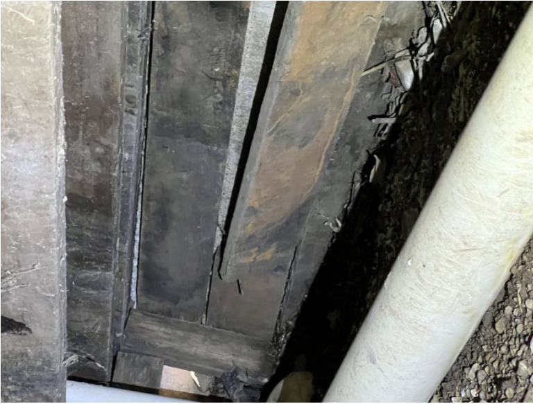
Image comments: Formwork still in position
