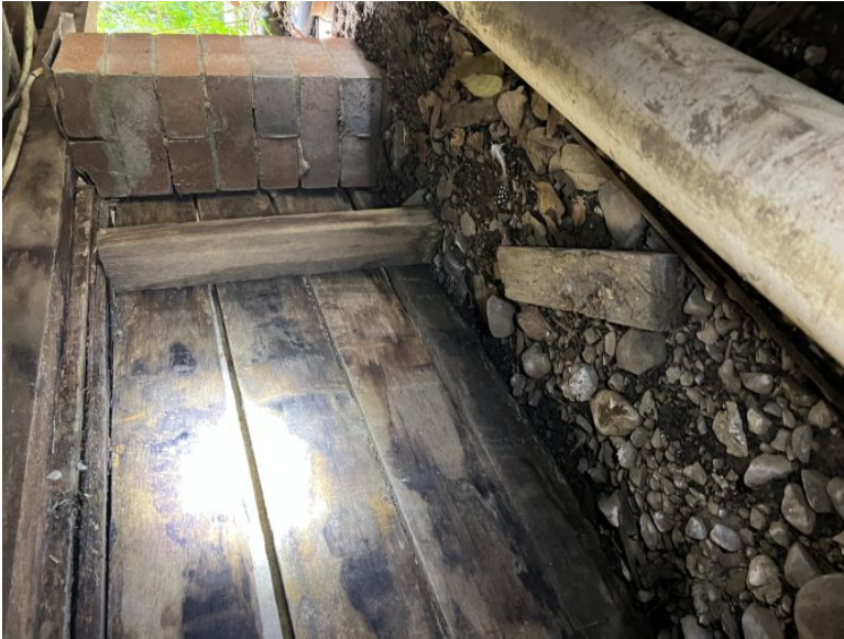
Image comments: Formwork still in position
