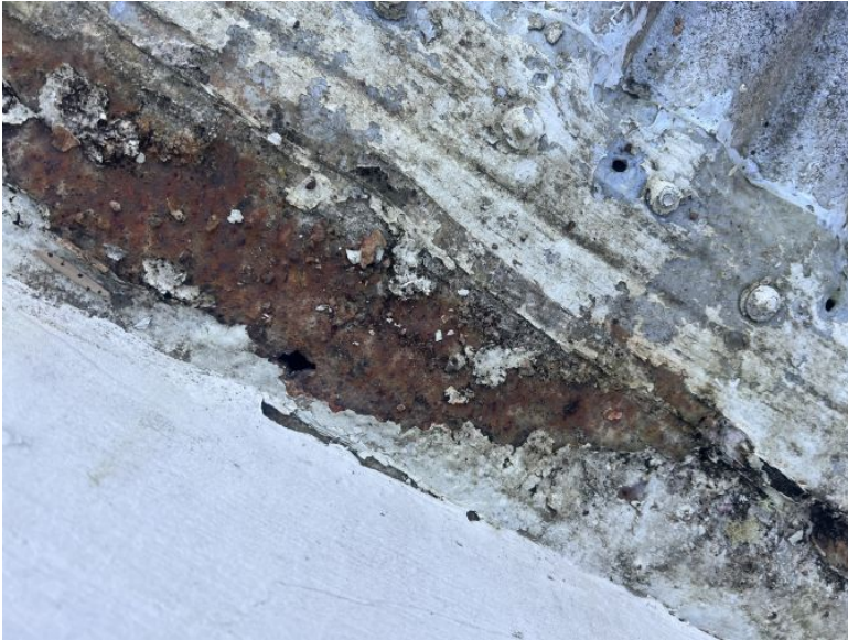
Image comments: Rust holes in apron flashing
